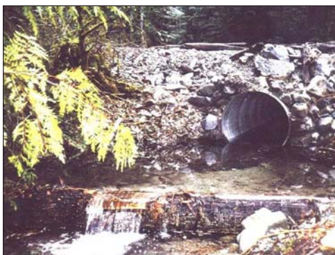
Posttreatment: Larger, sunken culvert with step-pool structure installed at culvert outlet.
